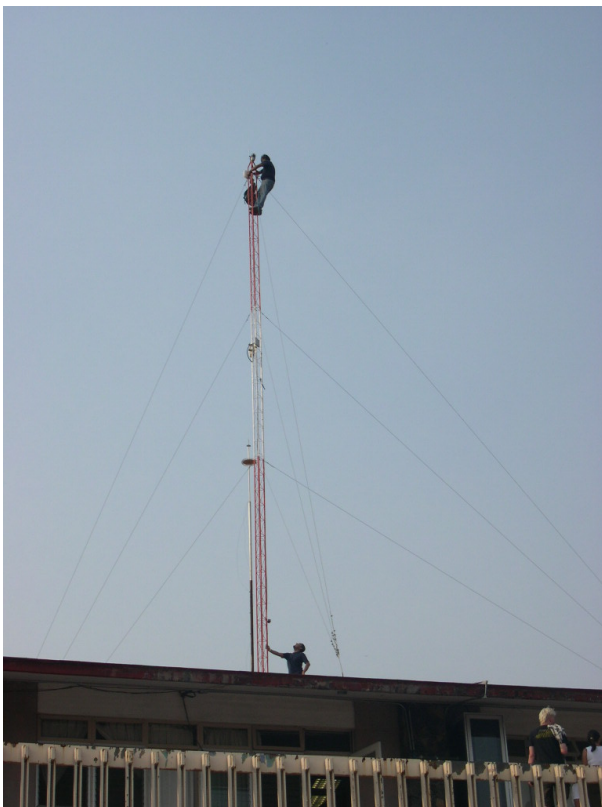
Direct line of sight to uplink, from a 30–40m high point
